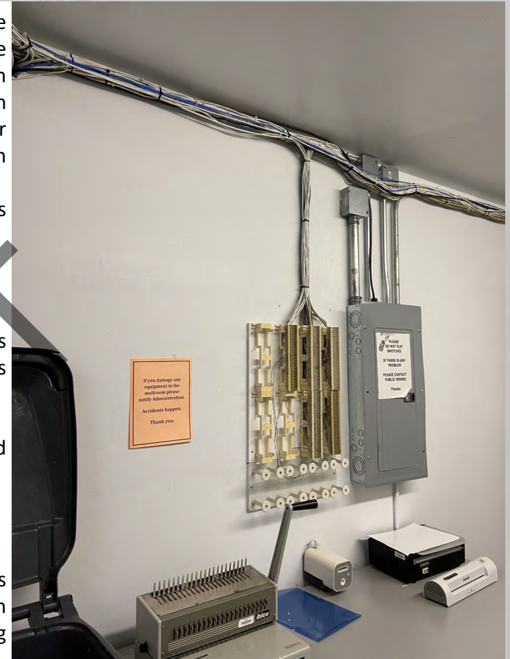
Figure 8-3. Exposed wiring in City Hall
