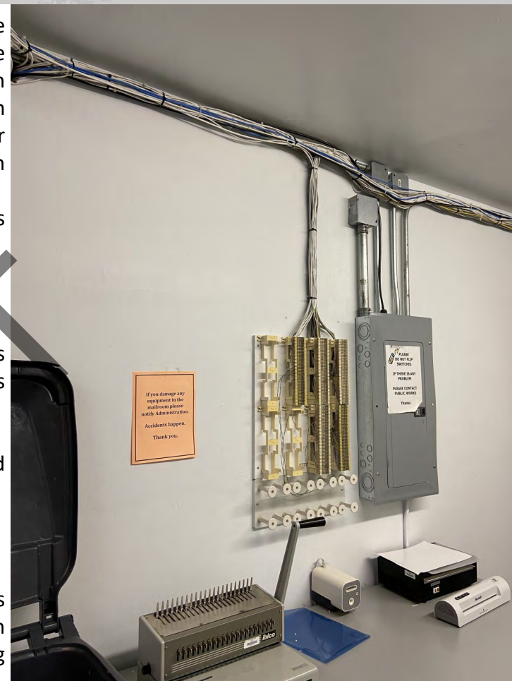
Figure 8-3. Exposed wiring in City Hall
