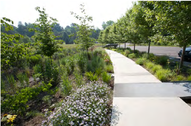
Figure 60. Bio-swales, similar to drainage ditches, utilize selected vegetation to filter and slow down stormwater runoff prior to its drainage into the water shed. These bio-swales can be designed using native vegetation adapted to the area, requiring minimal maintenance.
