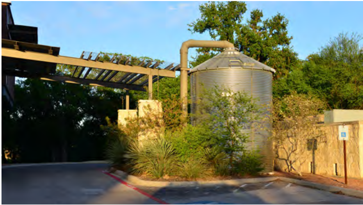
Figure 62. Rainwater harvesting should be considered during the development of future pavilions. The above example captures rainwater from a pavilion roof top and stores it in a 5,000 tank for use in irrigation of the park landscape.
