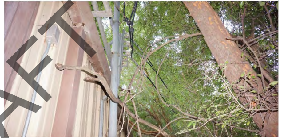
Figure 8-2. Above: Vegetation around Cart Barn power source. Below the structural members of the roof are showing major corrosion.
